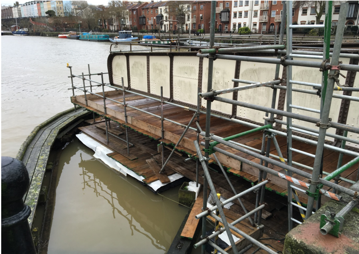
Floating Pontoon scaffolding underneath cantilevered unsupported end of bridge.
