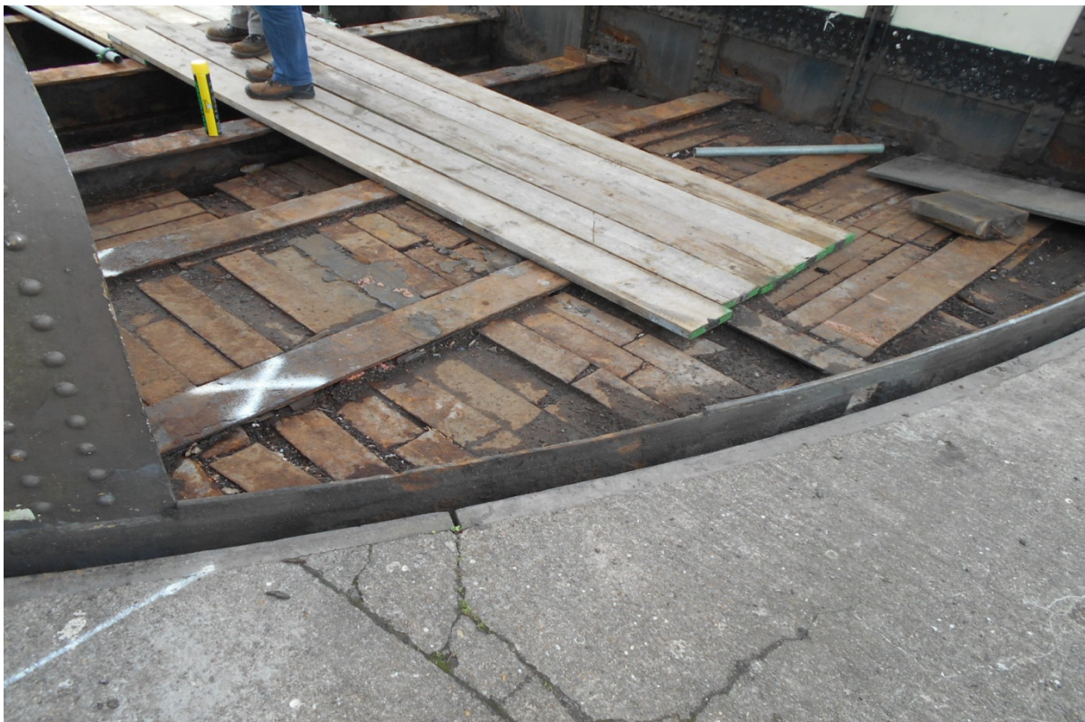
Pig Iron Counterweights exposed at Kentledge end of Bridge before removal
