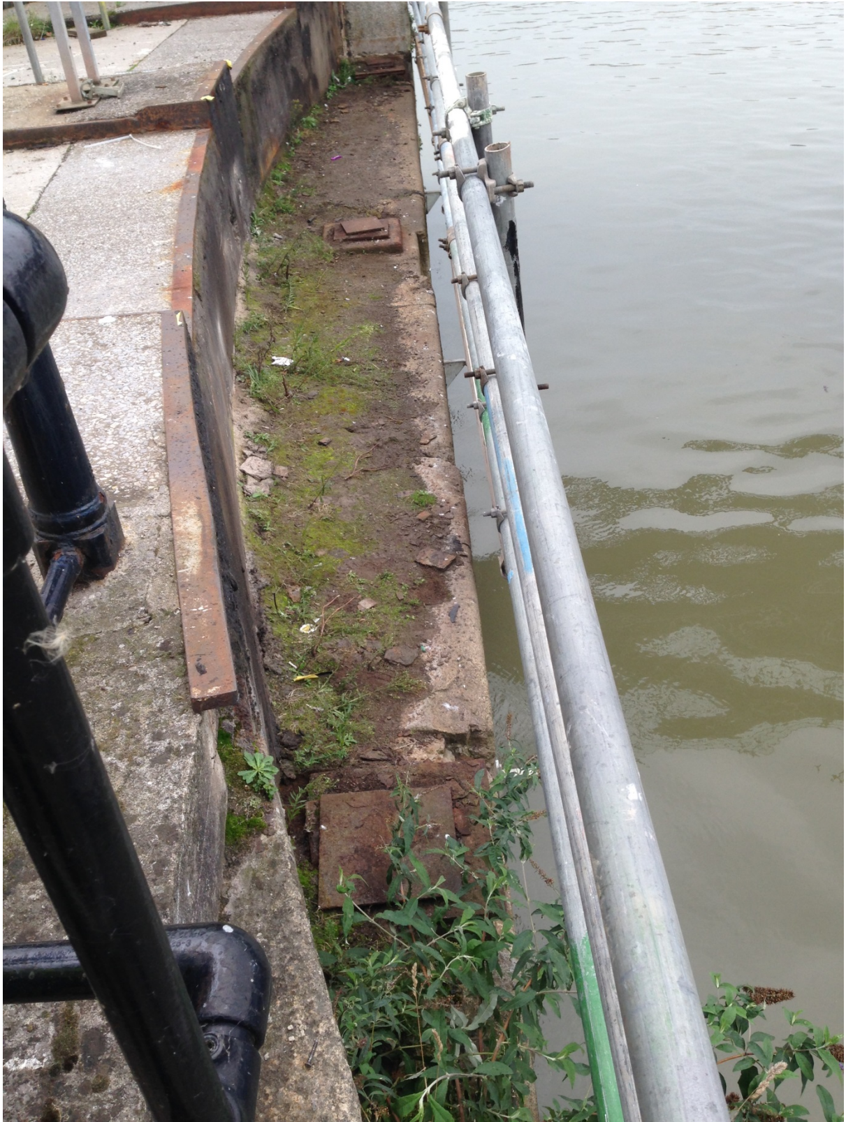
Condition of South Abutment Shelf and bearing Pads, currently being refurbished
