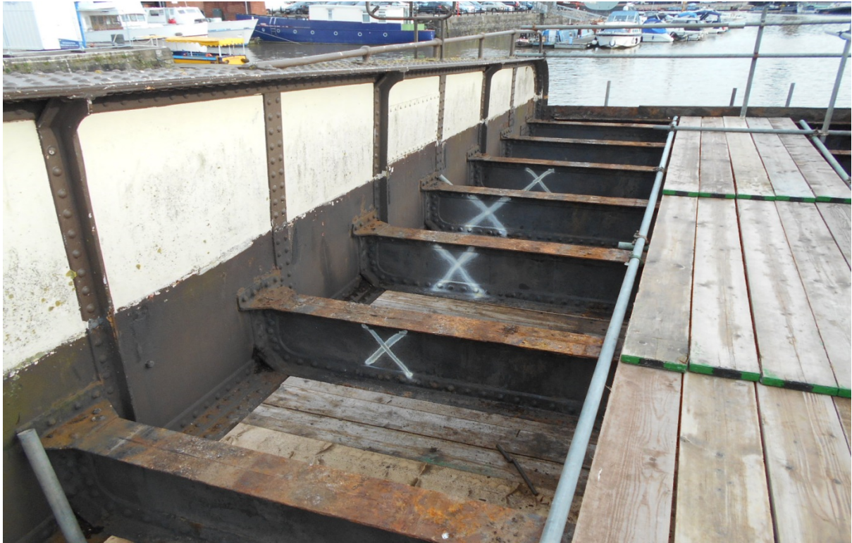
Further marked cross beams due for removal and replacement
